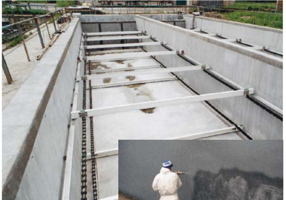
Spray application VANDEX POLYCEM Z
